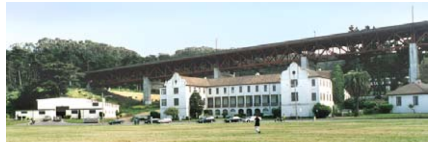
Figure 6: Presidio Viaduct looking northeast from the stables
