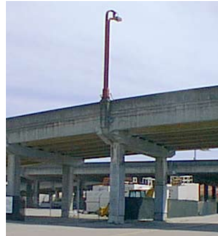
Figure 8: Light standard and guardrail
