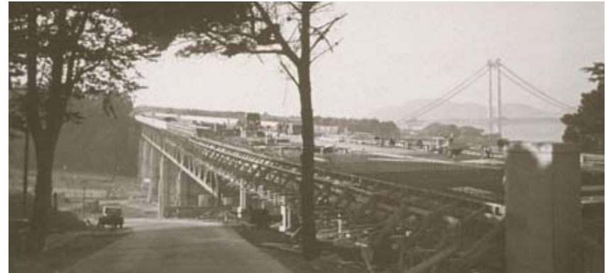
Figure 5: Presidio Viaduct under construction looking west from Lincoln Boulevard toward the stables area
