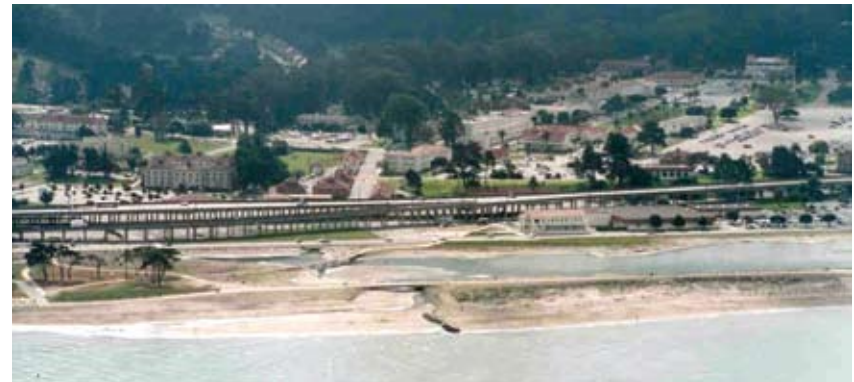
Figure 7: Marina Viaduct looking south from San Francisco Bay
